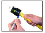
Verify the stab fitting is the correct size for the polyethylene (P.E.) pipe. Verify the SDR (or
