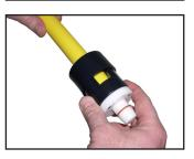
Stab pipe completely into fitting so that the mark on the pipe is within 1/8" from the fitting entrance.
